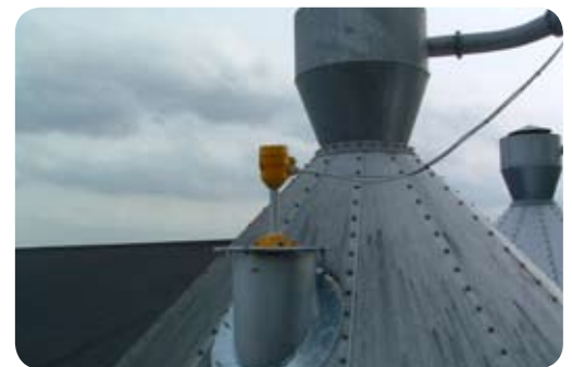
Ultrasonic sensors measure the feed level in the silos and the information are sent regularly to the production system using FältCom MIIPS® terminals.
